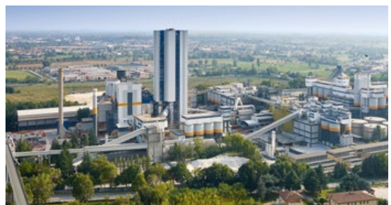
Production facility → Rezzato Cement Plant
